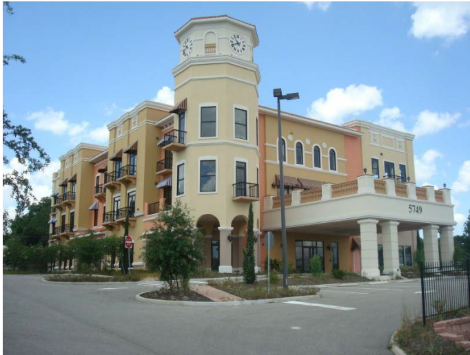
Westgate Dr Office Building in Orlando, Florida.
