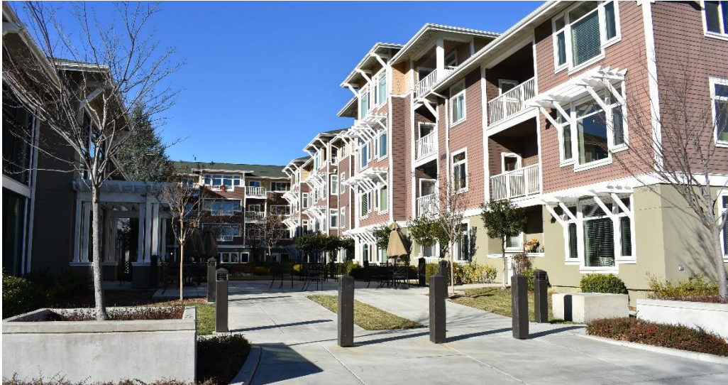
Figure 7 Shared Community Courtyard, Winters, California
