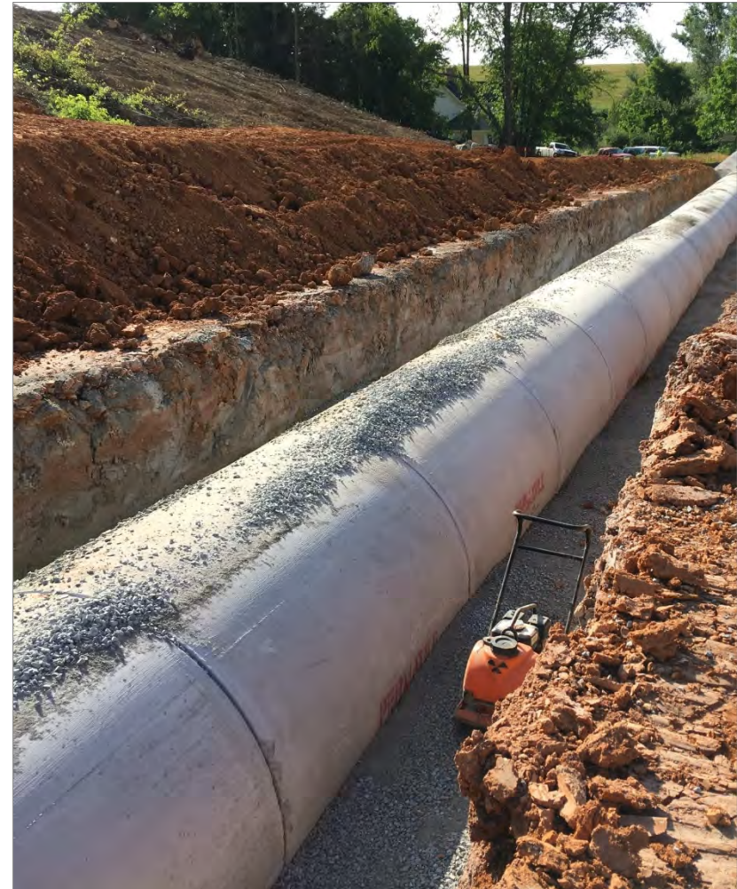
Concrete Drainage Pipeline
