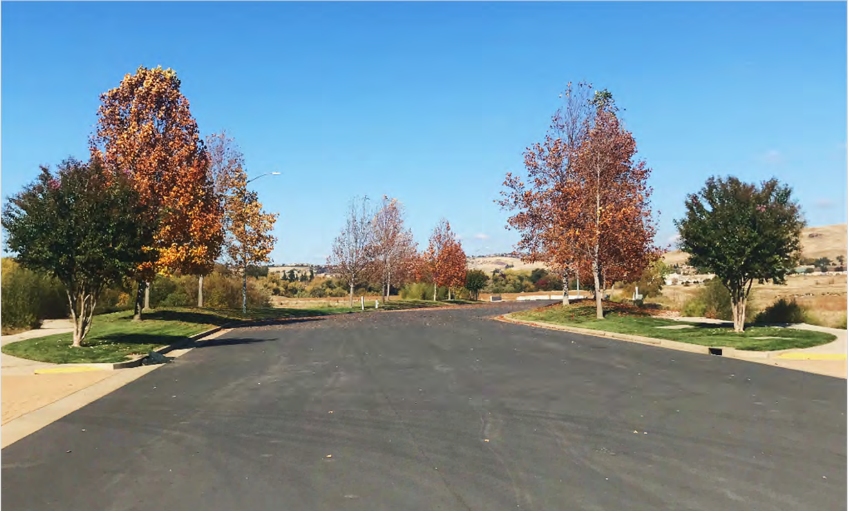
Previously Constructed Section of Carson Crossing Drive on the Southern Portion of the GED Site Looking North
