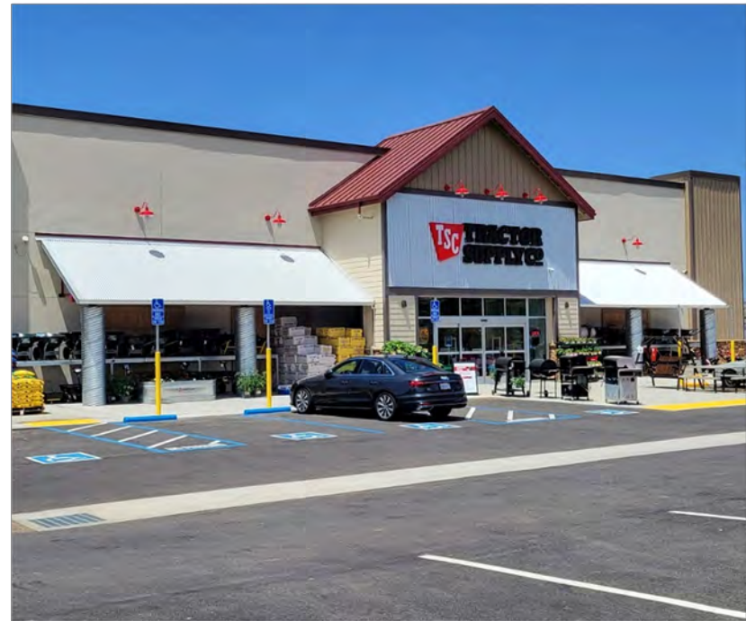
Commercial – GED Existing Tractor Supply Company
