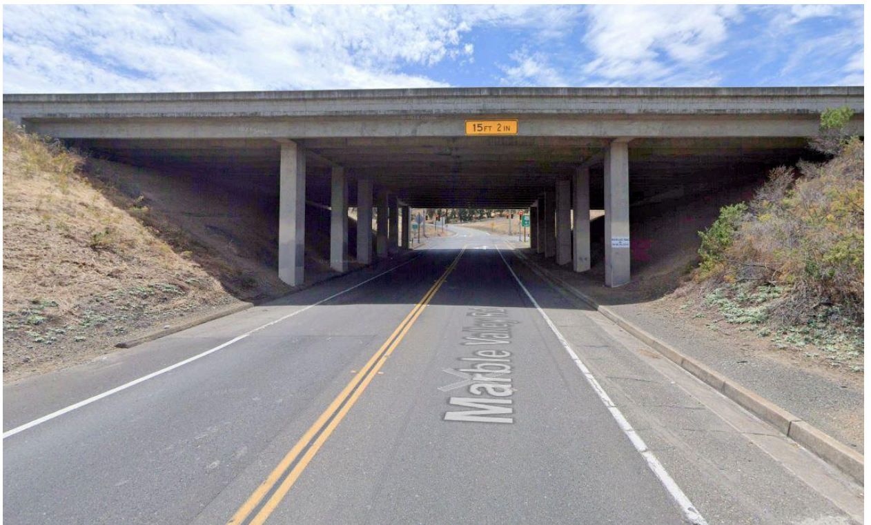
Bass Lake Road/Marble Valley Road US50 2-lane underpass - south view
