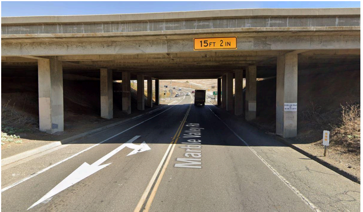
Bass Lake Road/Marble Valley Road US50 2-lane underpass - north view
