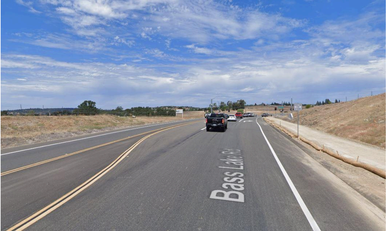
Northbound Bass Lake Rd approach to right turn lane at Country Club Drive - no turn signage
