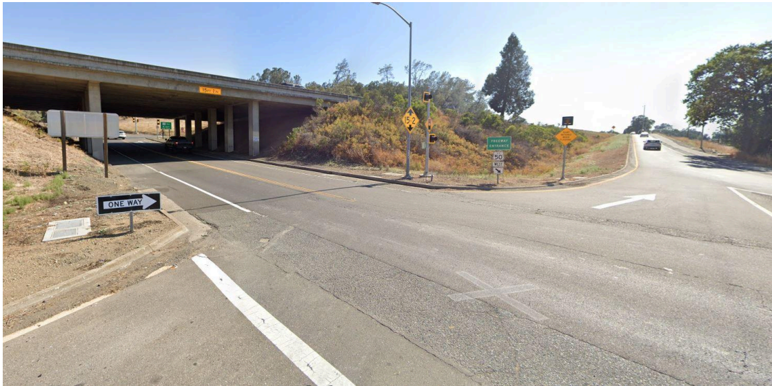
Westbound US50 Bass Lake Road off ramp with impeded visibility to the south
