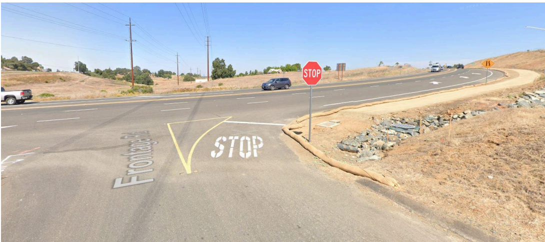
Old Country Club Drive/Frontage Road westbound approach to Bass Lake Road
