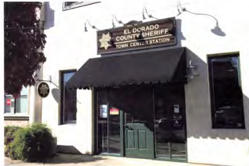
El Dorado County Sheriff Town Center Substation
