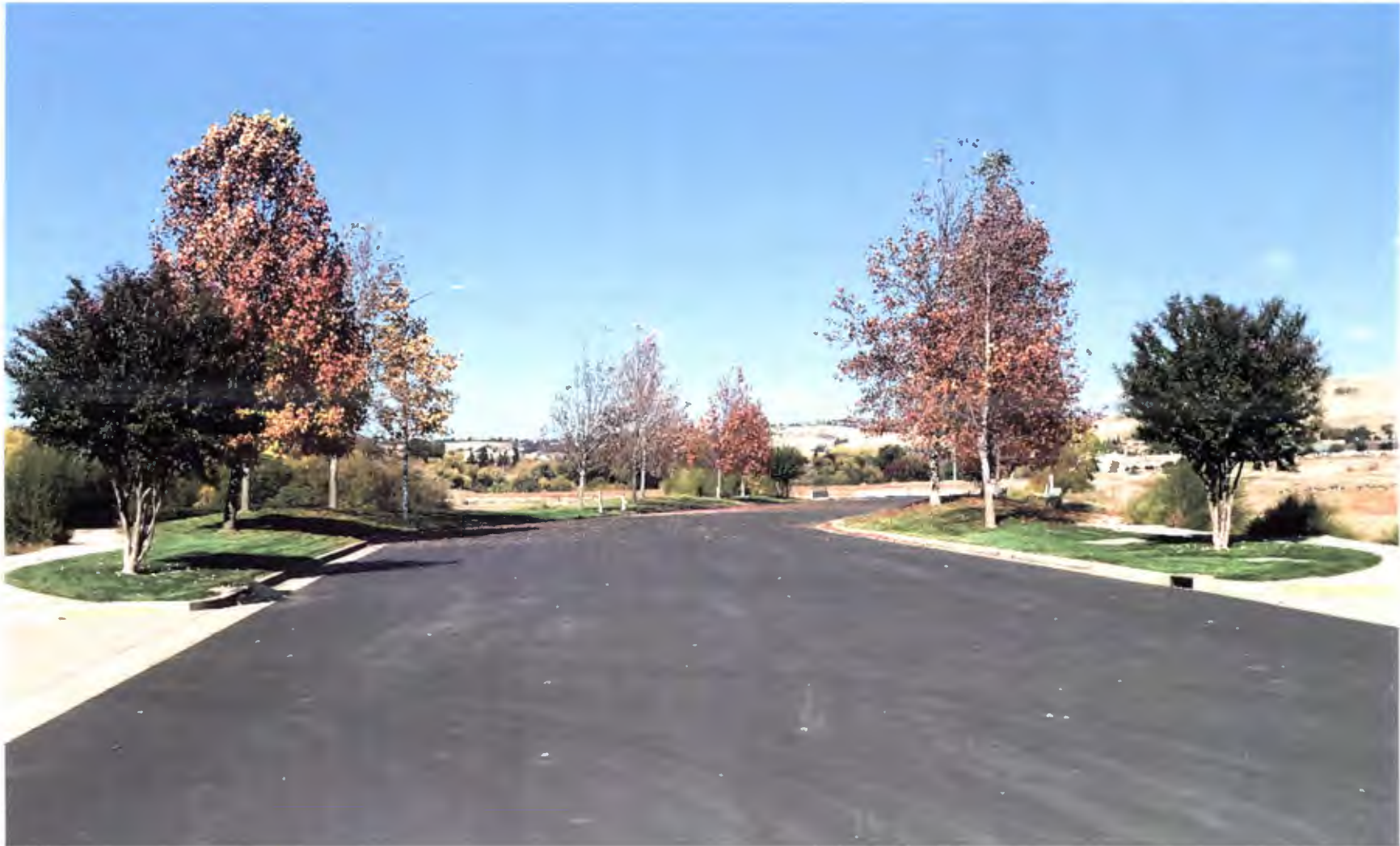
Previously Constructed Section of Carson Crossing Drive on the Southern Portion of the GED Site Looking North
