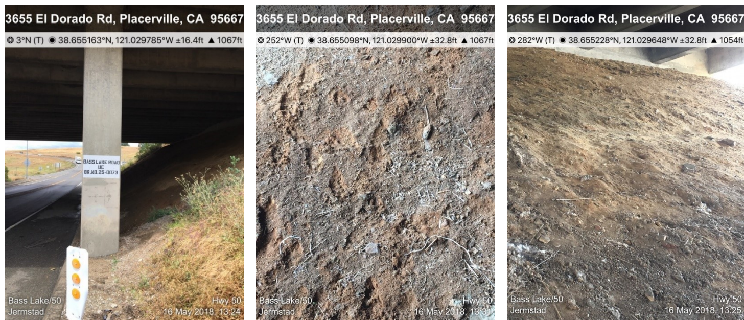
Figure 1. Bass Lake Rd Overcrossing (photo documented in 2018 and 2023)
