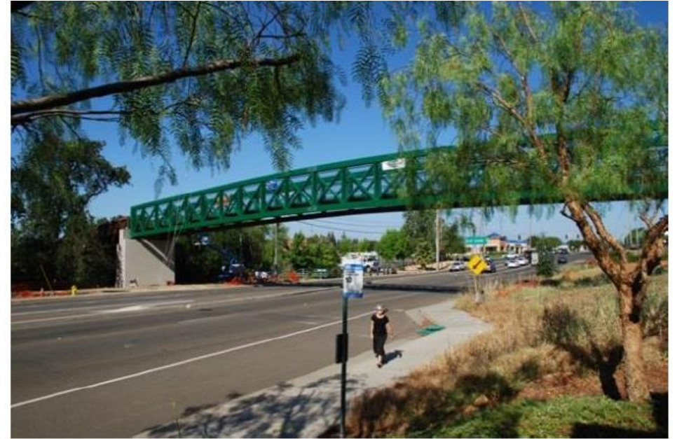
Pedestrian overcrossing at East Natoma Street and Blue Ravine Road, Folsom
